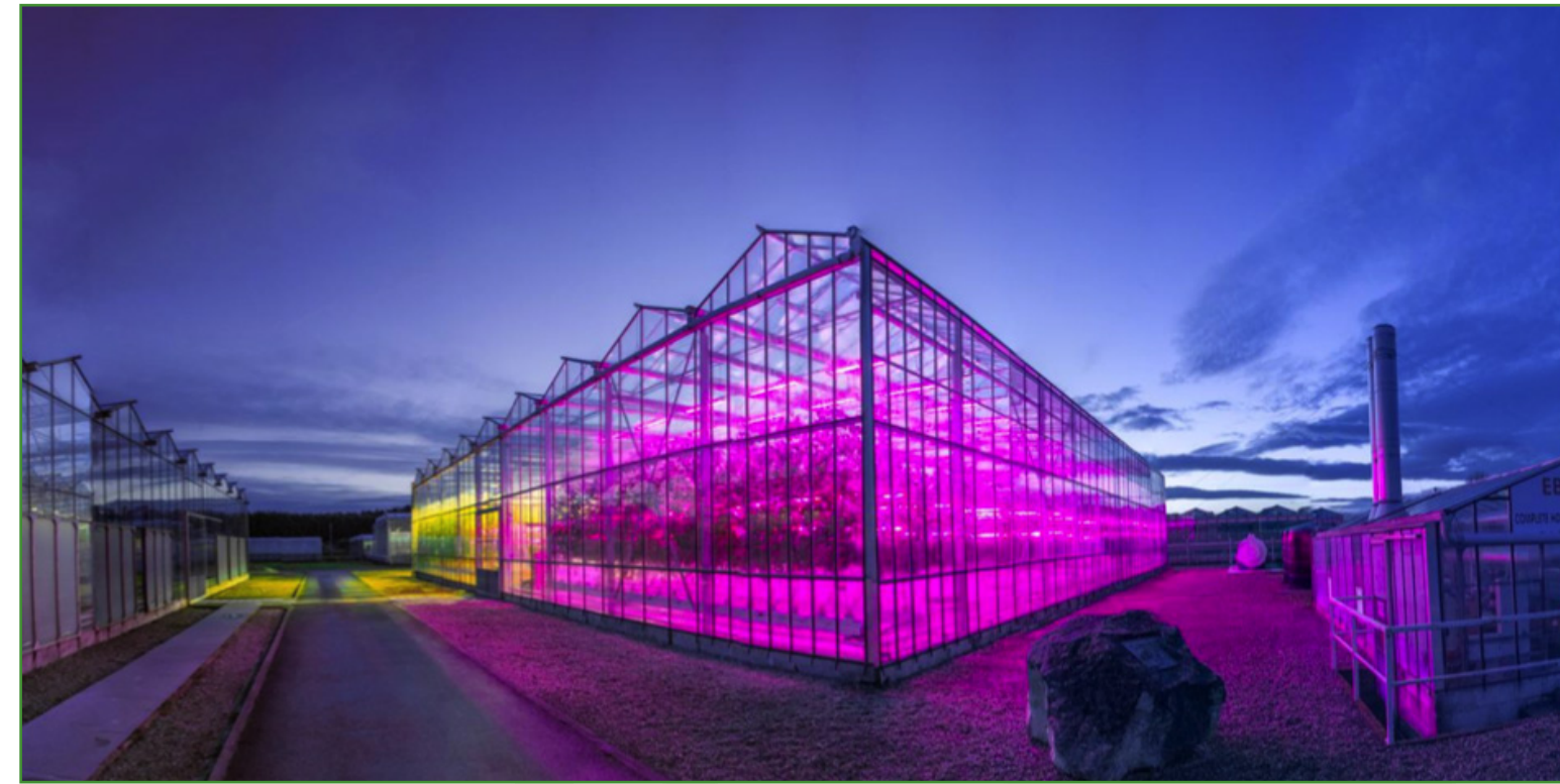
Figure 5: The LED4CROPS high wire glasshouse facility. This glasshouse contains four compartments each with a different lighting installation. Photograph provided by Philips
